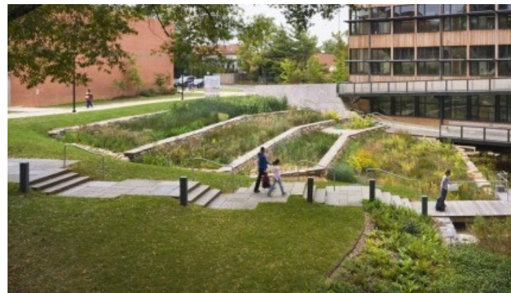
Constructed wetland suitable for shallower terraces
