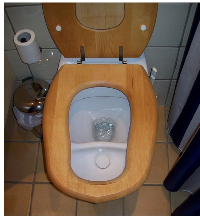
Urine diversion toilet flushing example
