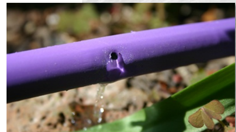
Drip Irrigation: must be differentiated by purple piping due to use of wastewater for irrigation
