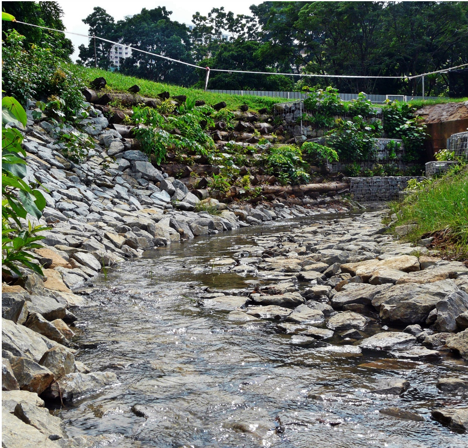
Successful bioengineering techniques implemented along riverbank
