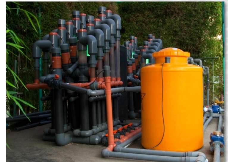
Unit capable of approximately 80 m 3 desal water / day
