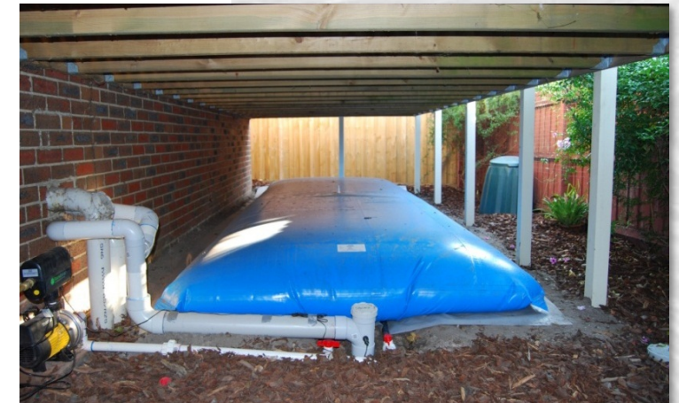
Reduce concrete encasement and place in 'bladders'
