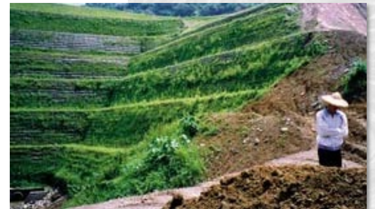
Revegetated geogrid over extreme slope condition
