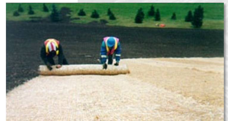
Erosion control mats over steep slopes
