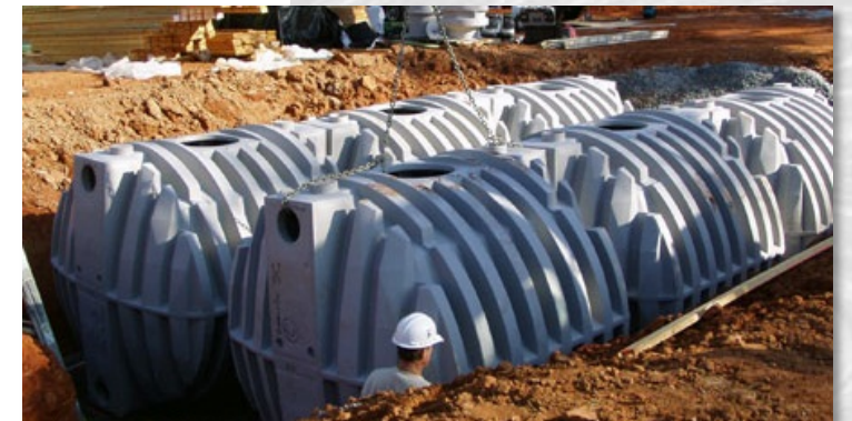
Polyethylene tank material safe for potable water
