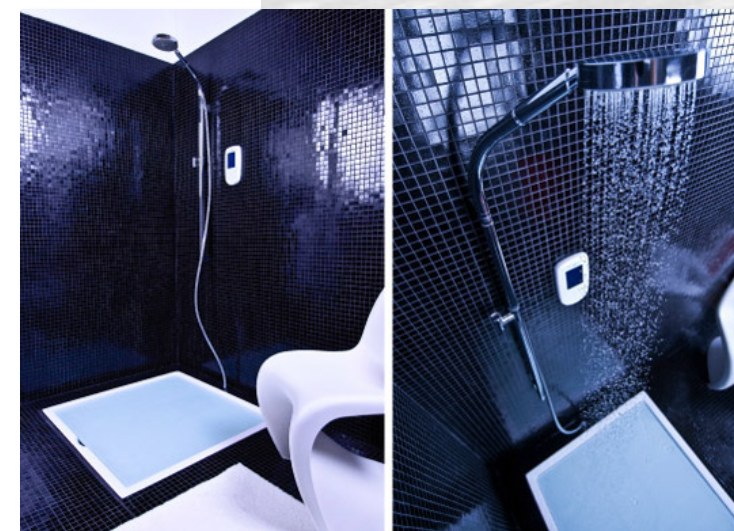
Eco-Shower filters, cleans, and recycles water
