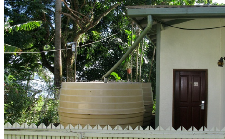
Storage can also occur aboveground in cisterns
