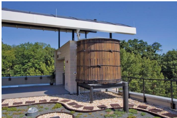
LEED Platinum Eco-Office collecting water from PV array
