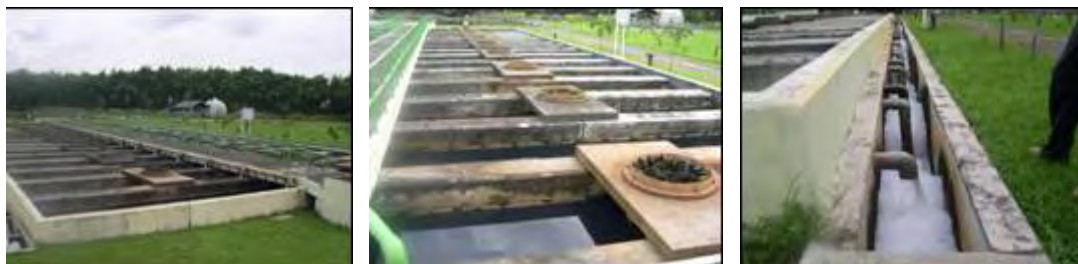
Photo by: Oni Hartono Date: November,29 '05 Location: WWTP Pulau Brayan Bengkel (Cemara) – Medan Remarks: (From left): UASB left part ; UASB right part ; outlet from UASB
