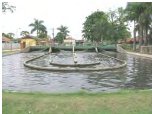
Photo by: Edzard Ruehe Date: October, 19 '05 Location: WWTP 'Tanah Tinggi' – Kota Tangerang Remarks: Aeration unit.
