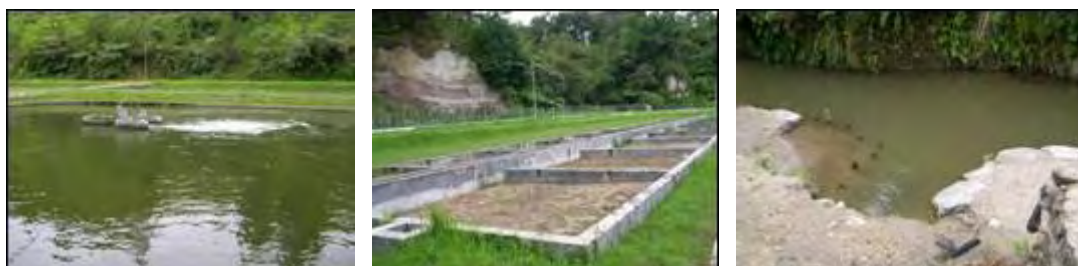
Photo by: Edzard Ruehe Date: December,05 '05 Location: WWTP Parapat - Ajibata Remarks: (From left): aerated pond ; sludge drying bed ; outlet to Sera-sera river
