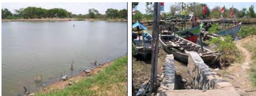
Photo by: Oni Hartono Date: October,06 '05 Location: WWTP Kesenden – Cirebon Remarks: (Left) Facultative pond (people fishing). (Right) Outlet from WWTP Kesenden goes to river /sea.
