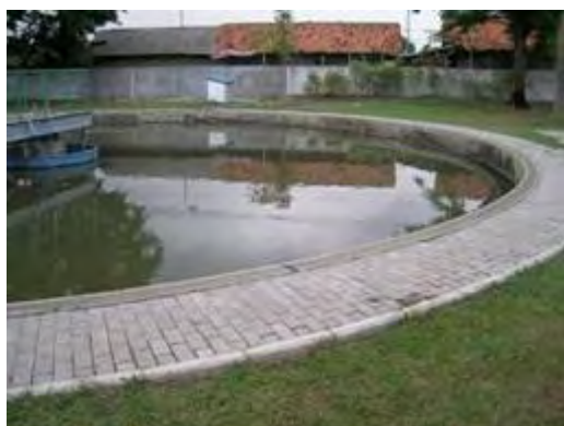
Photo by: Edzard Ruehe Date: October, 19 '05 Location: WWTP 'Tanah Tinggi' – Kota Tangerang Remarks: Clarifier tank with mechanical scraper.
