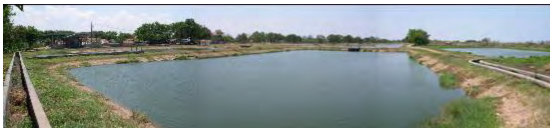
Photo by: Edzard Ruehe Date: October,06 '05 Location: WWTP Kesenden – Cirebon Remarks: Aerated pond (without aerator)
