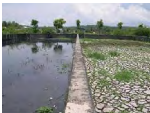
Photo by: Edzard Ruehe Date: October,25 '05 Location: WWTP Sewon – Bantul - Yogyakarta Remarks: (left) sludge drying bed, (right) outlet from WWTP.
