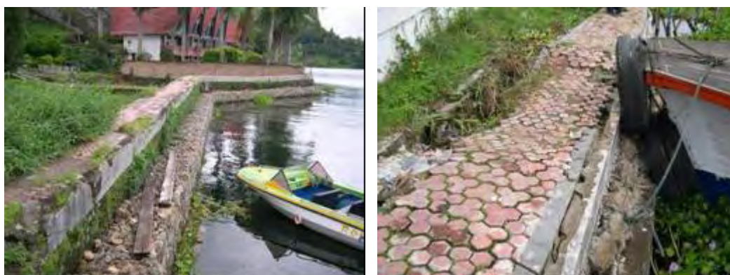
Photo by: Edzard Ruehe Date: December,05 '05 Location: Parapat Remarks: (Left): sewerage pipe line (right): pipe bed is used by boats.
