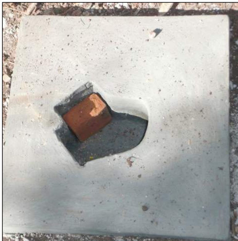
Figure 8-7: Control box or 'Y'-junction (SHAW/Spit, 2012)
