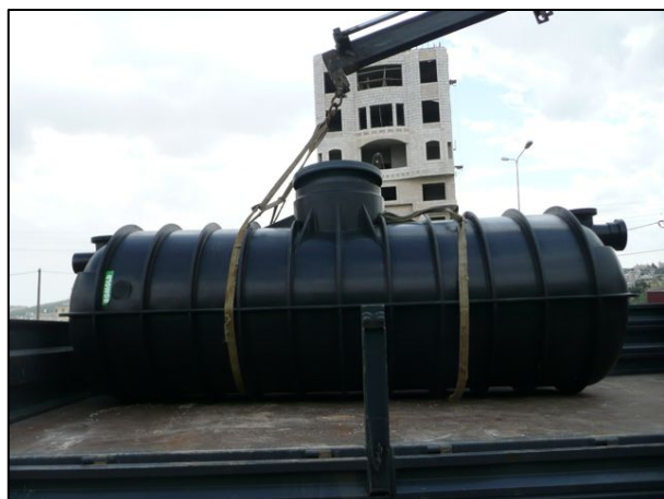
Figure 8-101: HDPE Septic Tank (UNICEF/Spit, 2012)
