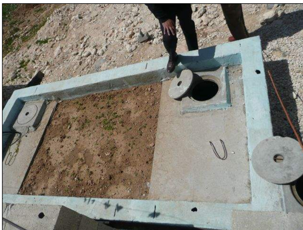
Figure 8-174: Household grey water anaerobic upflow filter (UNICEF/Spit, 2012)
