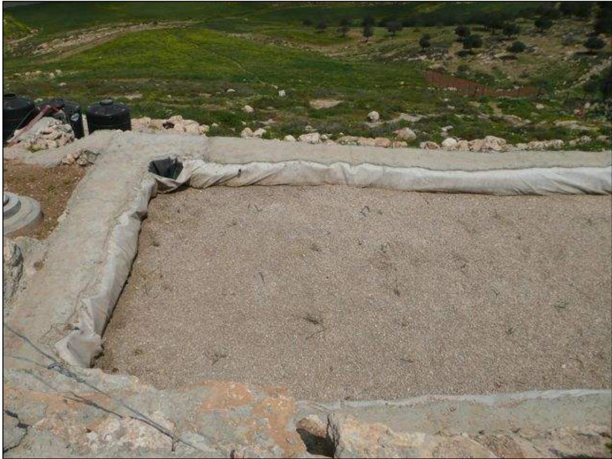
Figure 8-185: Village grey water anaerobic upflow filter (UNICEF/Spit, 2012)
