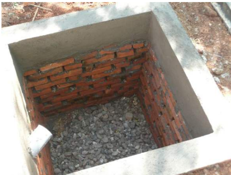
Figure 8-6: Detail pit (SHAW/Spit, Indonesia 2012)
