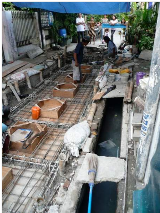
Figure 10-6: ABR under construction (Spit, Surabaya, 2011)
