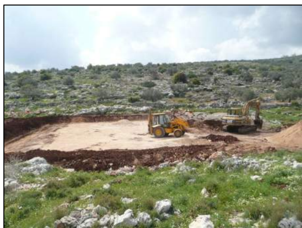
Figure 9-7: Constructed wetland under construction
