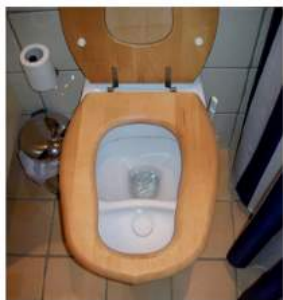
Urine diversion toilet flushing example
