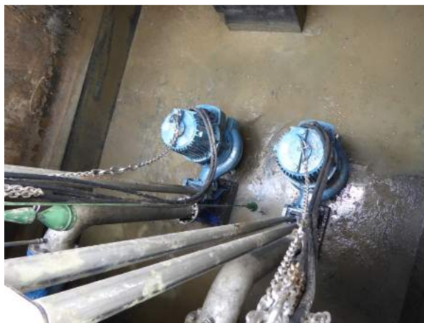
Figure 6: Cleaned pump sump
