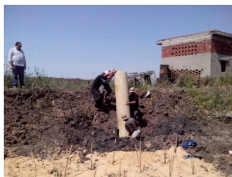
Photo 3 & 4: construction of pilot CW. A layer of 10 cm white sand was placed in the pond bottom. (Photos: Frank van Dien)
