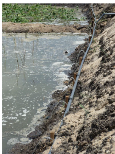
Photo 5, 6 & 7: Pilot CW water inlet structure; water outlet structure and overview of the CW. (Photos: Peter G.M. van der Heijden)
