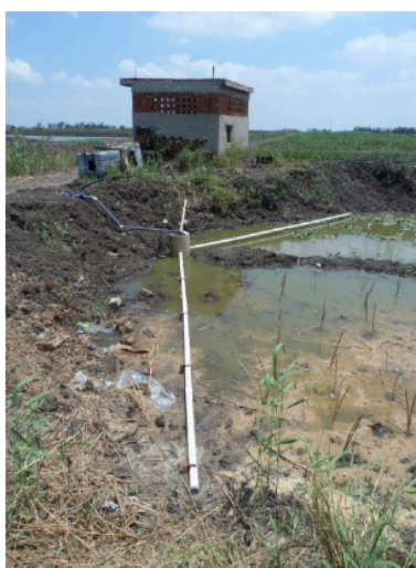
Photo 5, 6 & 7: Pilot CW water inlet structure; water outlet structure and overview of the CW. (Photos: Peter G.M. van der Heijden)
