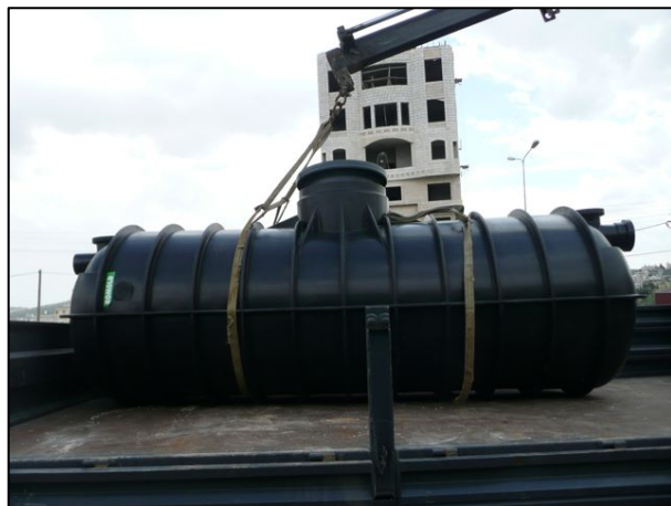
Figure 14: HDPE Septic Tank (Spit, 2012)
