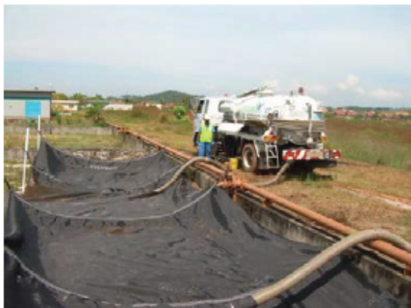
Figure 19: Sludge transfer station by geotubes
