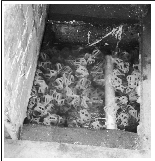
Figure 11: Plastic Filter Media (Sasse, 1998)
