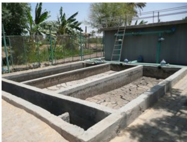
Figure 25: Sedimentation tank (right) and sludge drying bed (left)
