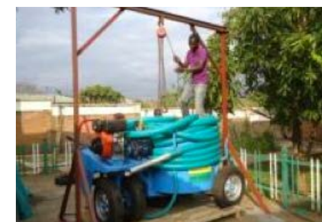
Figure 47: Lifting the Vacutug for assembly using lifting gear.
