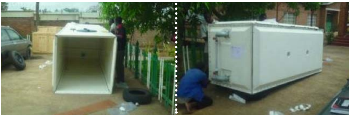
Assembling the tank took 4 people almost 7 hours .
