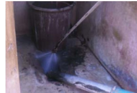
Figure 75: Fluidising is an essential part of pit emptying – including fishing out of rubbish from the now softer sludge and the pumping out the sludge.
