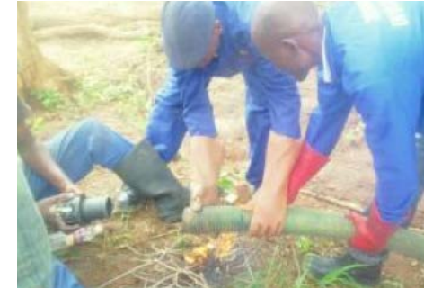
Figure 77: Heating the hose to fit the Camlock.
