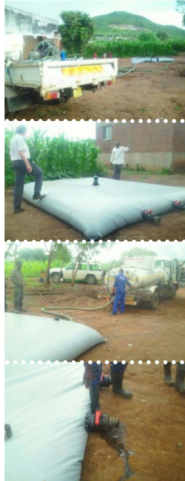
Figure 79: Operating the bladder.
