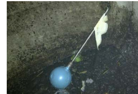
Figure 36: Jammed ball valve.
