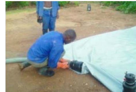
Figure 78: Fitting Camlock.
