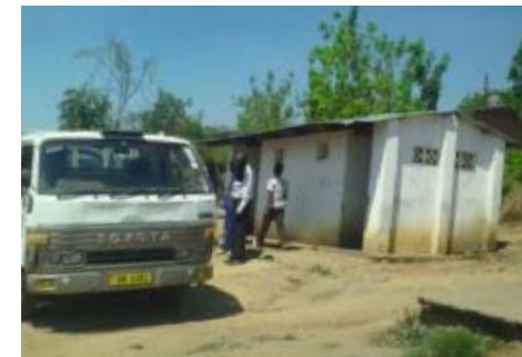
Figure 25: The original length of 3" suction pipe supplied is 15m, and is too short to access many toilets.
