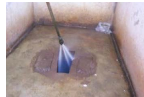
Figure 76: The fluidiser - with the pointed nozzle is essential for the safe cleaning process.
