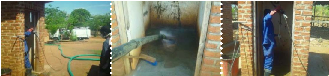
Figure 26: The length of the suction pipe is now 30 m (2 x 15 m) so we can access more toilets – while the suction is still very good. We are able to fill the tank in about 4 minutes.
