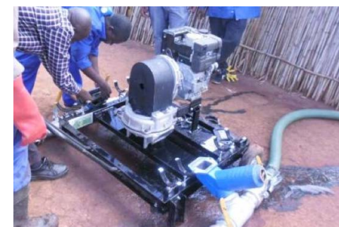
Figure 65: Dismantling, cleaning and reassembly of the 2 ports takes 30 minutes.
