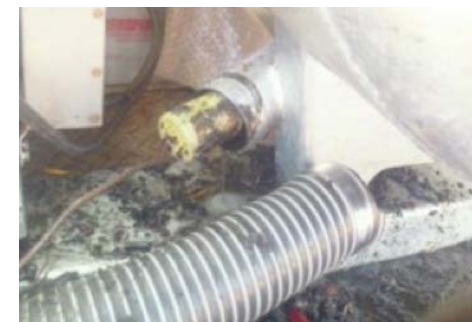
Figure 34: Items blocking discharge port include ARV bottles which escape fishing process – and we counted 4 bottles.
