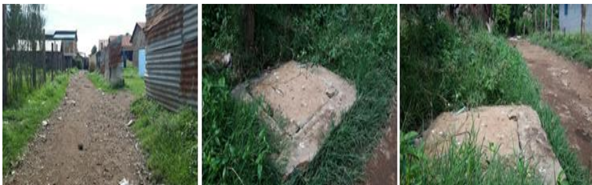
Figure 22: One of the Lateral Lines Implemented during the Pilot Project Expanding Sewerage Infrastructure into Manyatta A Settlement
