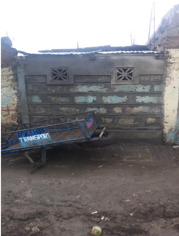
Figure 27: Ablution Block in Nairobi Informal Settlement as an Example for Kisumu
