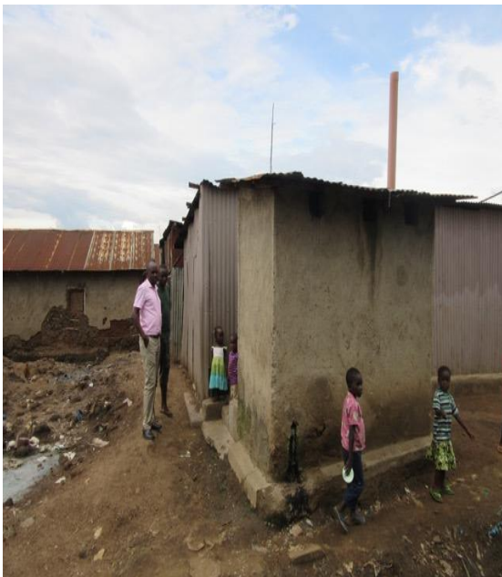
Figure 5: Typical Shared Toilet Cum Shower Facility
