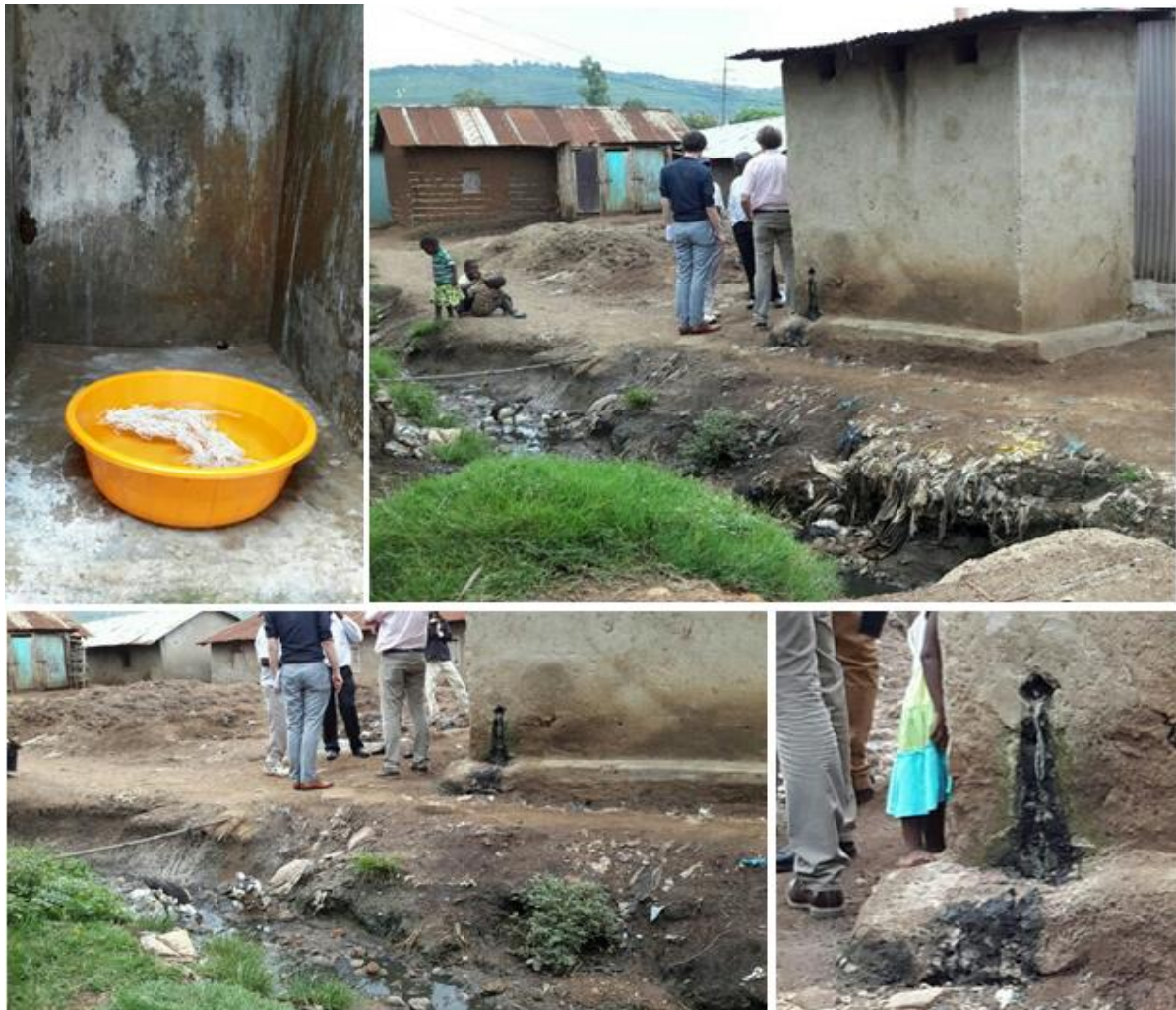
Figure 18: An Example of a Combined Pit Latrine and Bathroom in Obunga Informal Settlement that is Competing for Space with a Public Passageway due to Lack of Land
