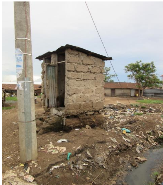
Figure 6: Typical Latrine: Emptied at Night into the Ditch
