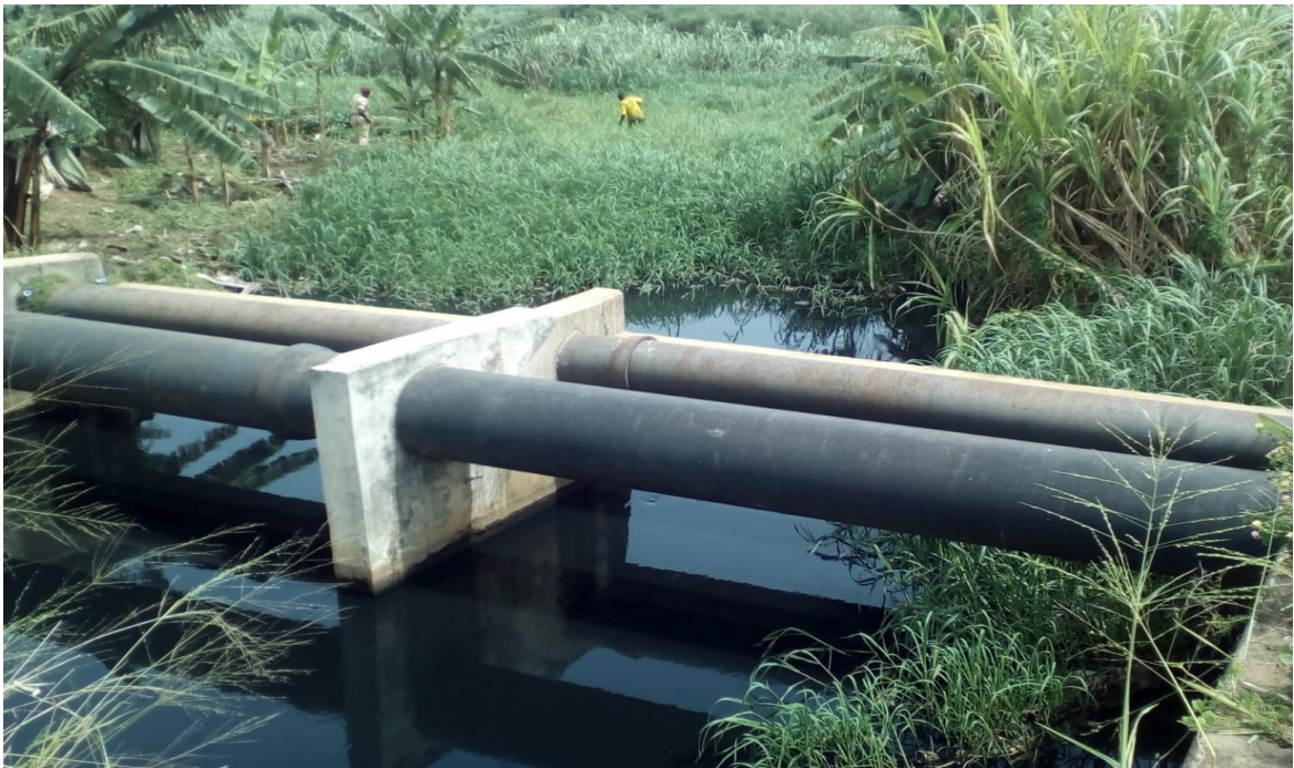
Figure 29: Dark Coloured Wastewater after Passing through the Existing Nakivubo Wetland
