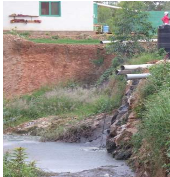
Figure 8: Discharge of Untreated Effluent Mechanical Sludge Dewatering Device
