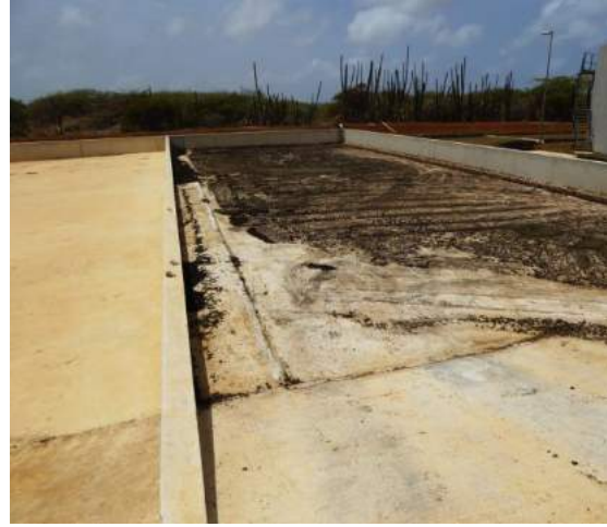
Figure 55: Sludge drying in open concrete beds (Photo: Jan Spit, Bonaire 2015)
