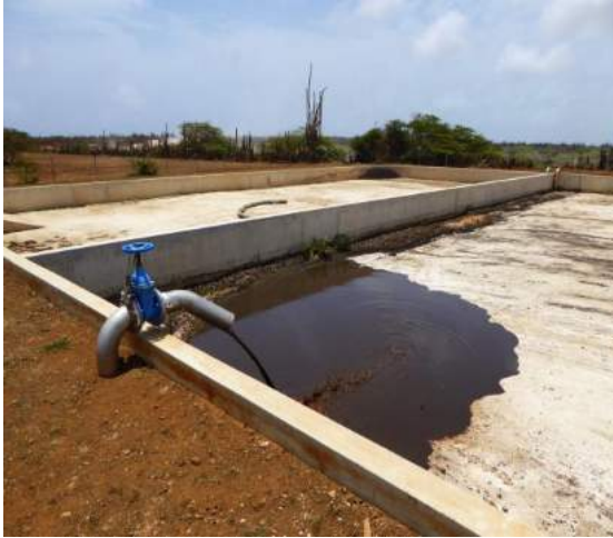
Figure 54: Sludge drying in open concrete beds (Photo: Jan Spit, Bonaire 2015)
