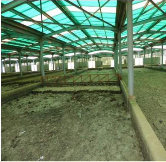
Figure 41: Sludge Drying Kampala
