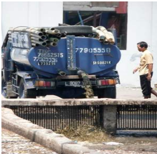
Figure 46: Sludge Reception with Screen in Surabaya, Indonesia (Photo: Jan Spit, 2011)
