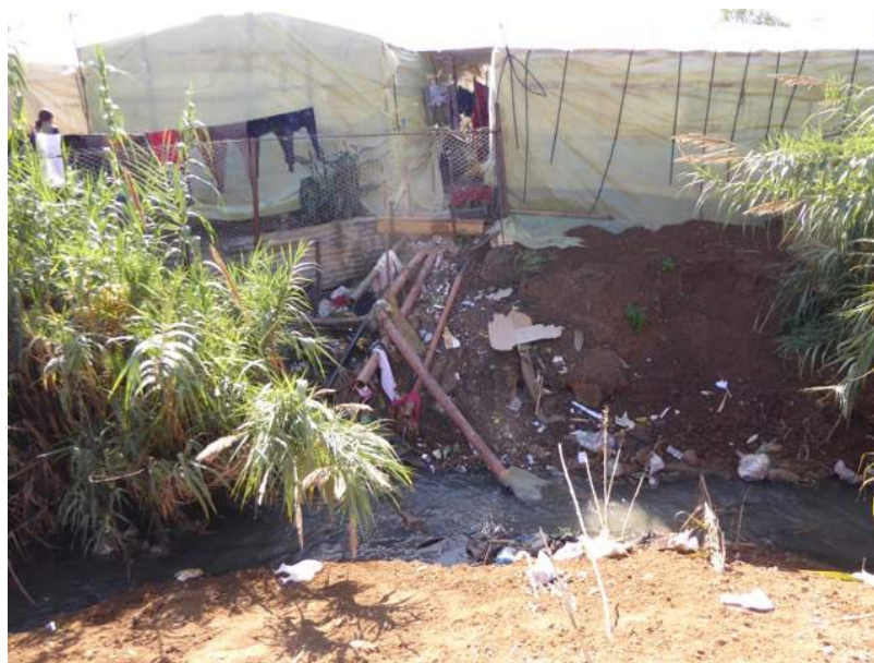
Figure 17: Discharge of black water into open channels
