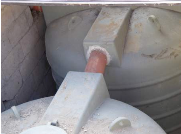
Figure 62: Connection pipe and tank using acrylic kit
