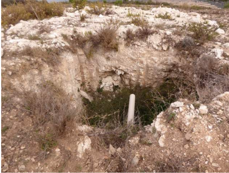
Figure 18: Discharge of black water in open (dry) pit
