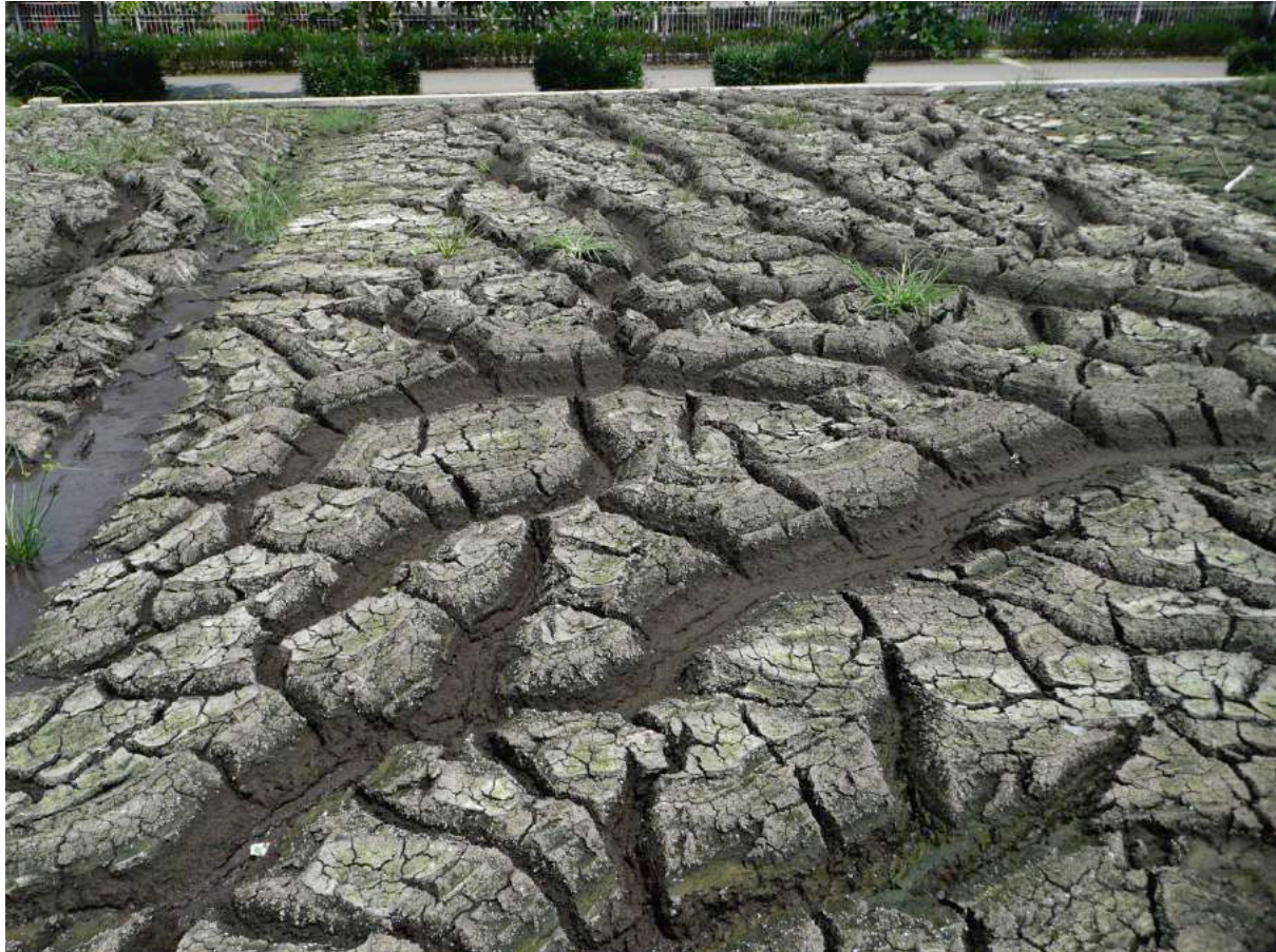
Figure 8: Sludge drying bed (Surabaya, 2010)
