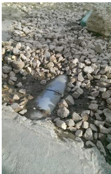
Figure 13: I ITS Zahle Mualqa 019: drainage pipes cut open every 15 cm to allow storm water infiltration
