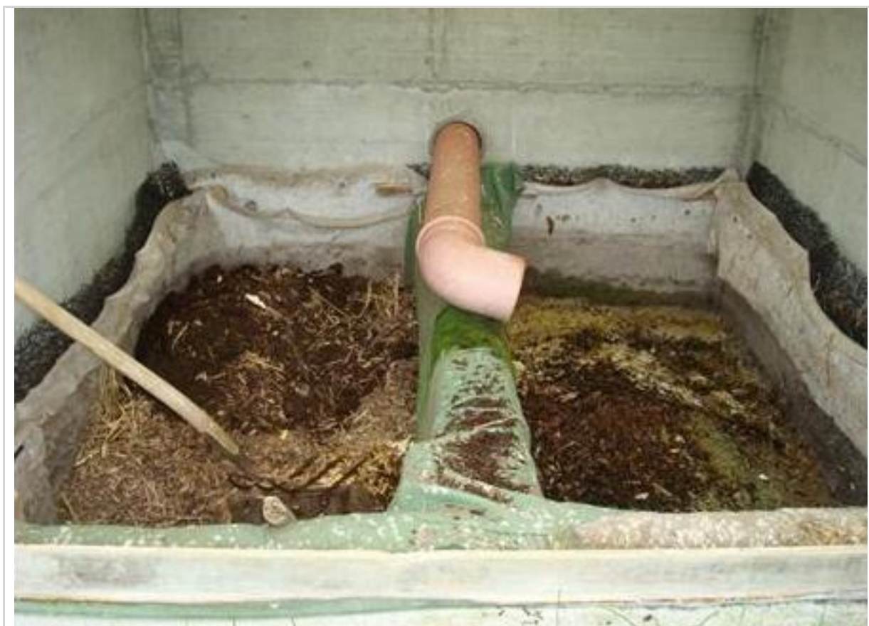
Operation of rottebehaelter (Staufer, 2010)
