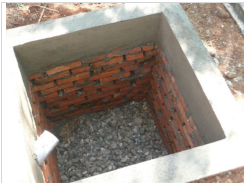
Honey comb brick work (WASTE, 2012)
