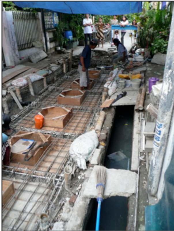
ABR under construction in Surabaya (WASTE, 2012)
